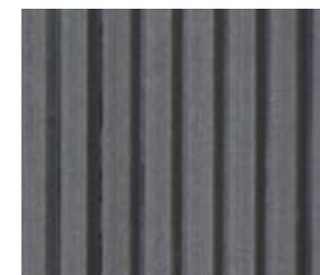
COARS RIBBED STRUCTURE
